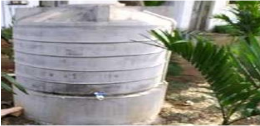
STP has 20000 Liters. For west water recycling
